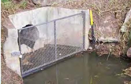
5. Wastes going to the environment can harm waters or wildlife. Screens can trap some of the solids, but not the liquids.
